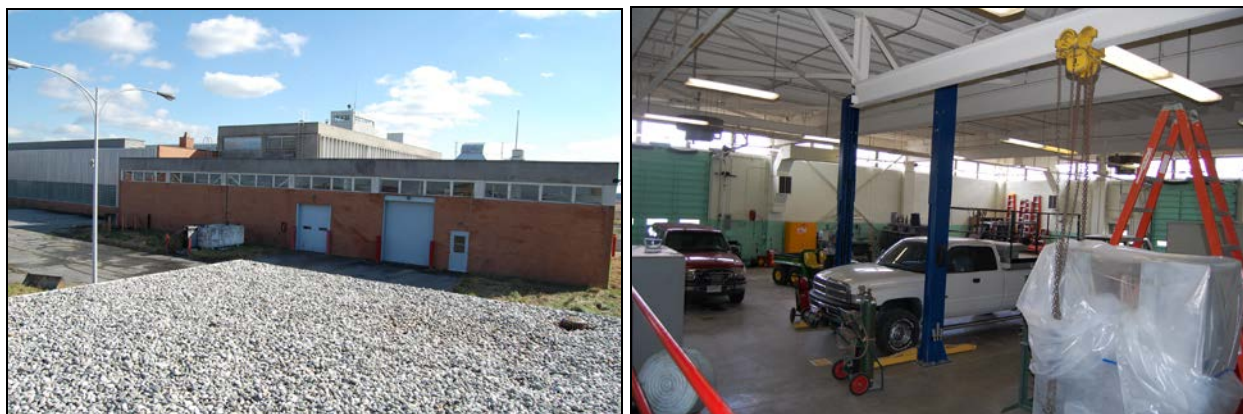
Figure 16. North elevation of one-story block (Site A), at left, and interior of garage with high banded windows (Site B), at right
