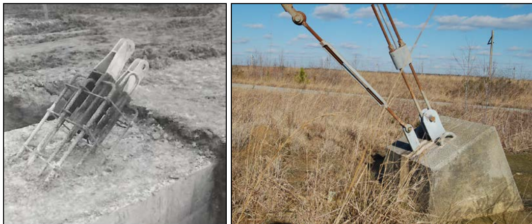
Figure 53. Curtain antenna H-4 (old numbering system) anchor, April 15, 1961, at left (source: VOA progress photographs file); anchor pier at log periodic antenna A-37, at right (both Site A)
