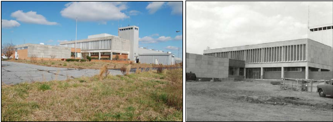
Figure 17. West front and south side elevations of transmitter building, at left, and same view of April 18, 1962 (both site A) (source: VOA progress photographs file)
