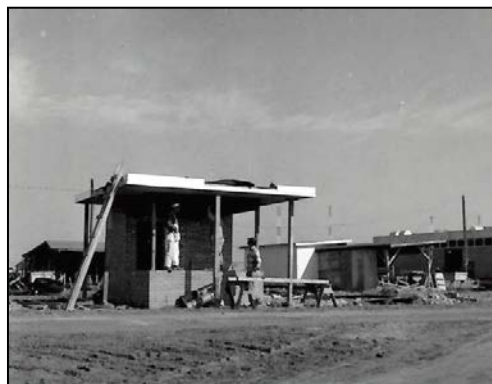
Figure 34. Site A guardhouse under construction, February 20, 1962 (source: VOA progress photographs file)
