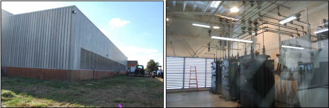
Figure 24. Louvered north side of building (Site A), at left, and transformer power vaults with louvers opening to north (Site B), at right
