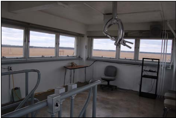
Figure 22. Tower observation room with hanging grip for searchlight (Site B )
