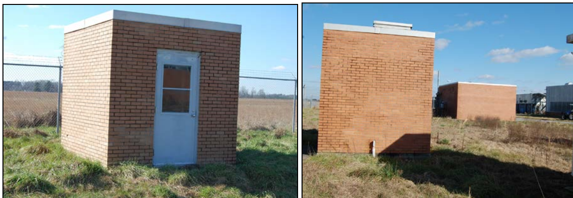
Figure 37. At left, well pumphouse 3; at right (from left to right), well pumphouse 2, generator building, and switchbay and transmitter building (both Site A)
