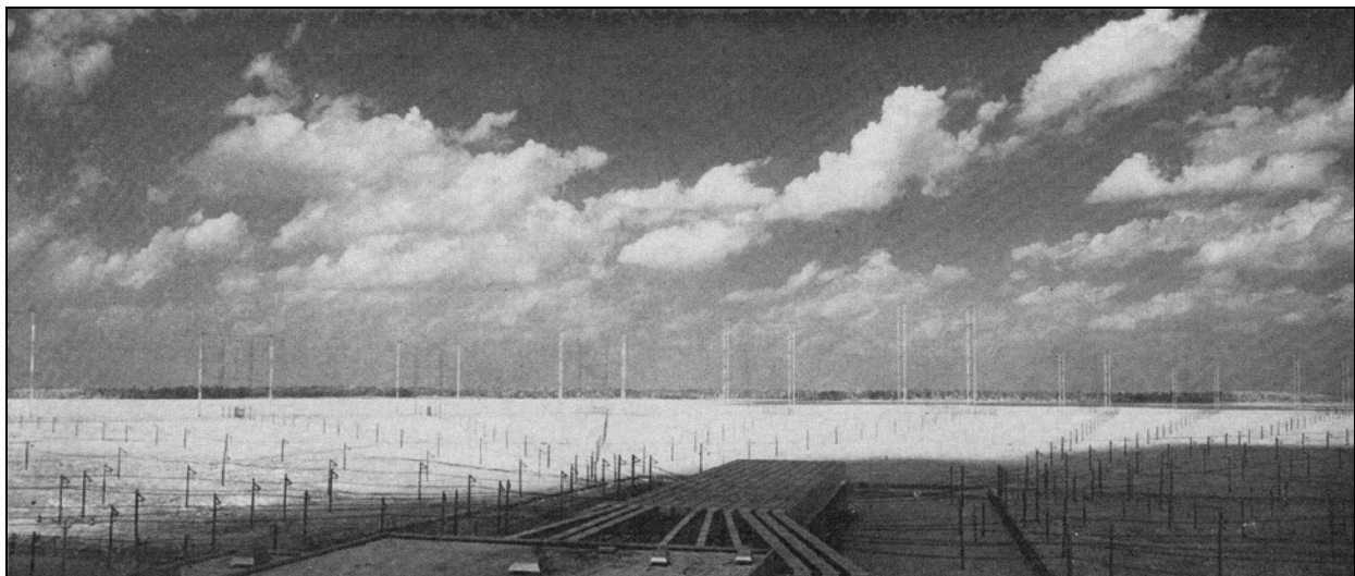
Figure 43. Site A antenna field with transmission building and switchbay in foreground (source: Rhine 1968:53)
