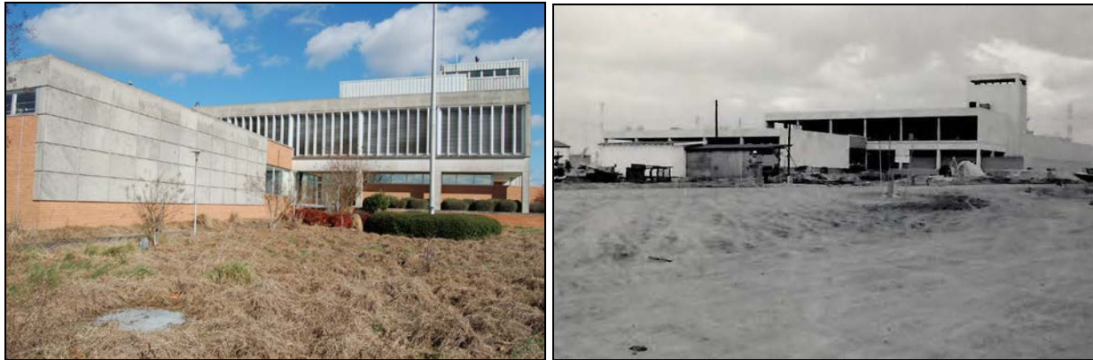
Figure 15. South elevation of one-story block, at left, and similar view of December 20, 1961, at right (both Site A) (source: VOA progress photographs file)
