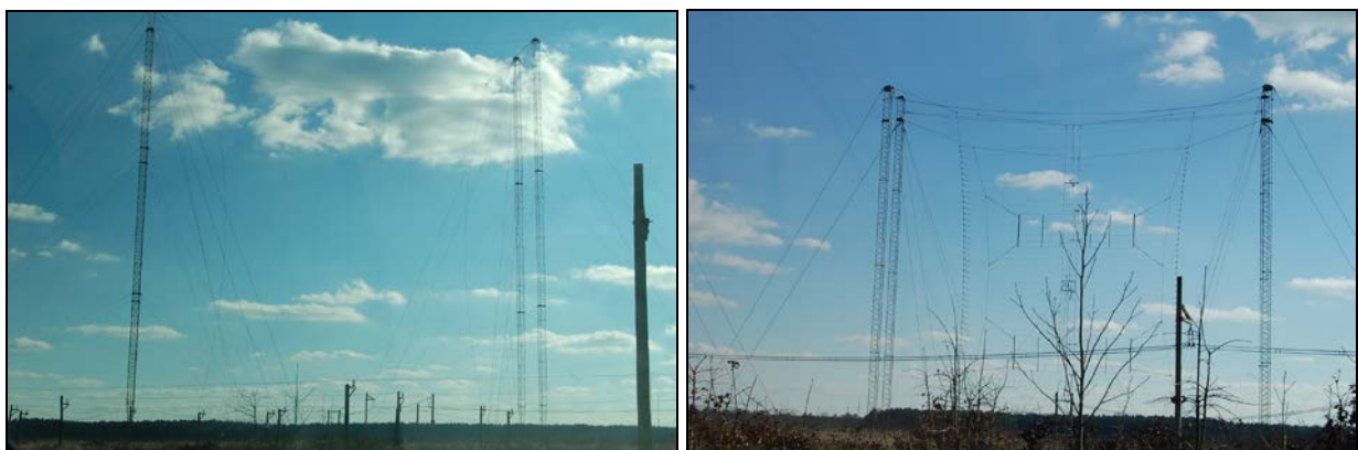
Figure 54. Dipole antenna AD-12B, at left, and dipole antenna AD-37, at right (both Site A)
