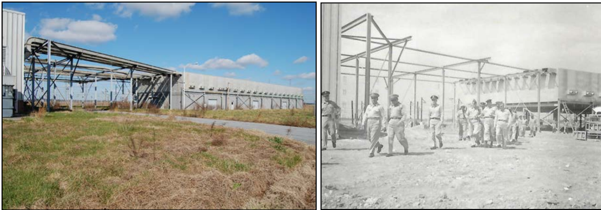
Figure 32. South side and west front elevations of switchbay connected to east rear of transmitter building by input conduits; same view, at right, including visitors from Fort Bragg War College, April 28, 1962 (both Site A) (source: VOA progress photographs file)
