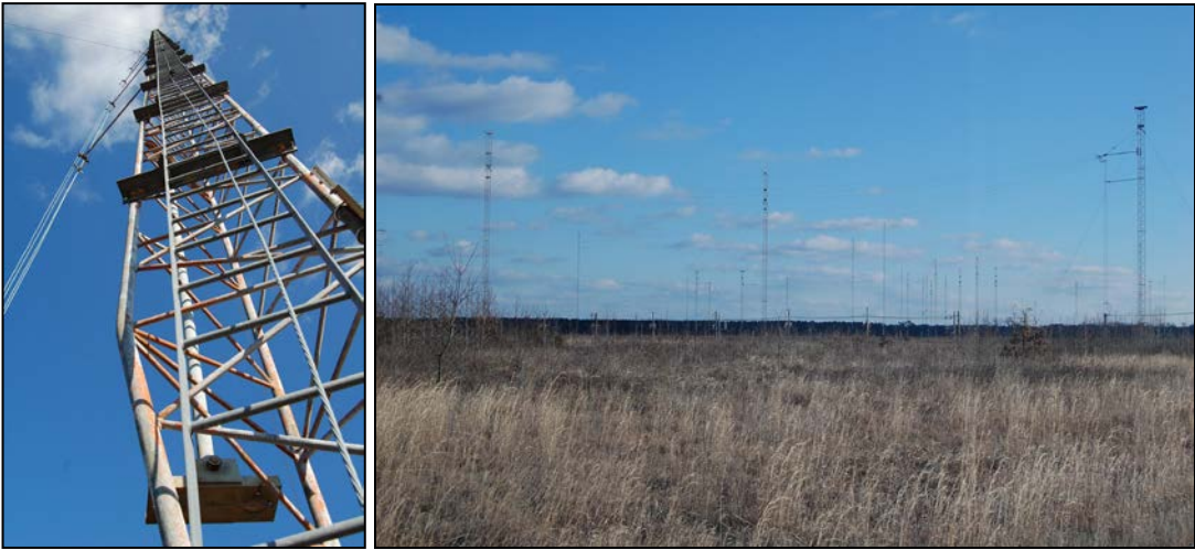
Figure 46. One of the towers of rhombic antenna A-01, at left; field of rhombic antennae along southern section of main service road south of antenna A-17, at right
