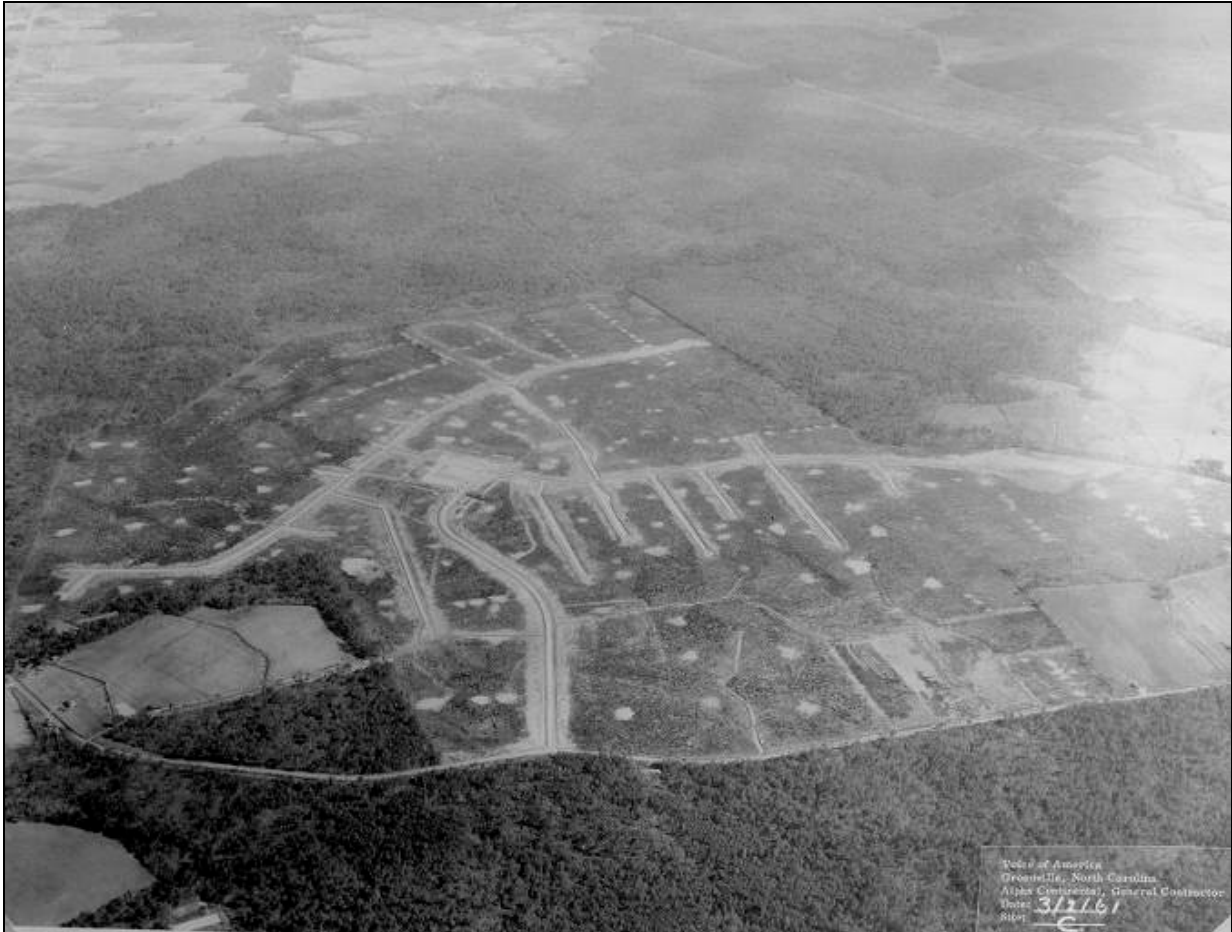
Figure 11. Aerial view of Site C cleared and ready for construction, March 2, 1961 (source: Greenville, NC Daily Reflector, May 3, 1961)
