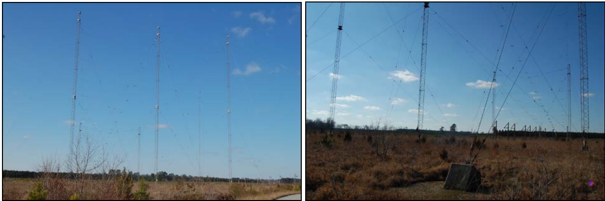
Figure 52. Log periodic antenna A-37 with, at left, all six support towers visible, three in foreground and three in distance (Site A)
