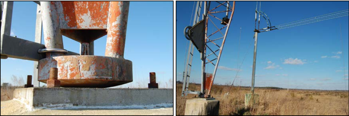
Figure 47. At left, base plate of one tower of rhombic antenna A-01 on anchor pier (note that tower is not affixed to ground); at right, concrete anchor pier and metal base plate of antenna A-01 with pulley for hauling parts
