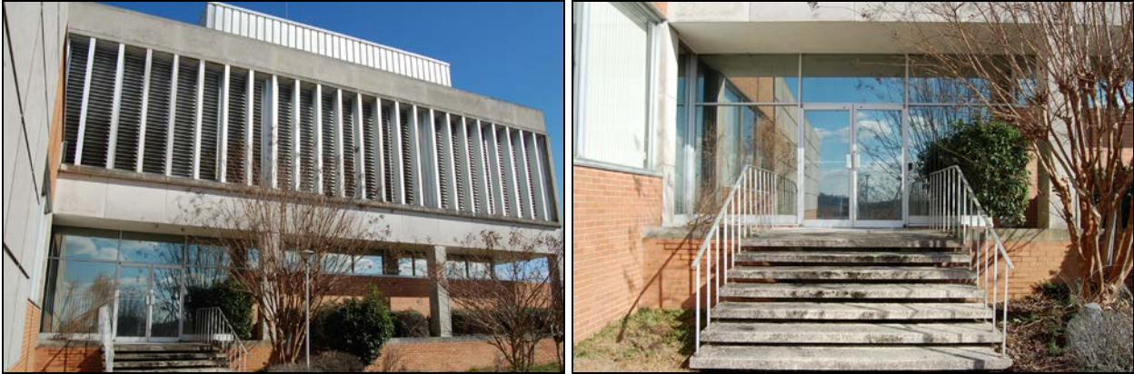
Figure 19. East front elevation of transmitter building with aluminum fins at cantilevered upper story, at left, and floating stair and lobby, at right (both Site A)
