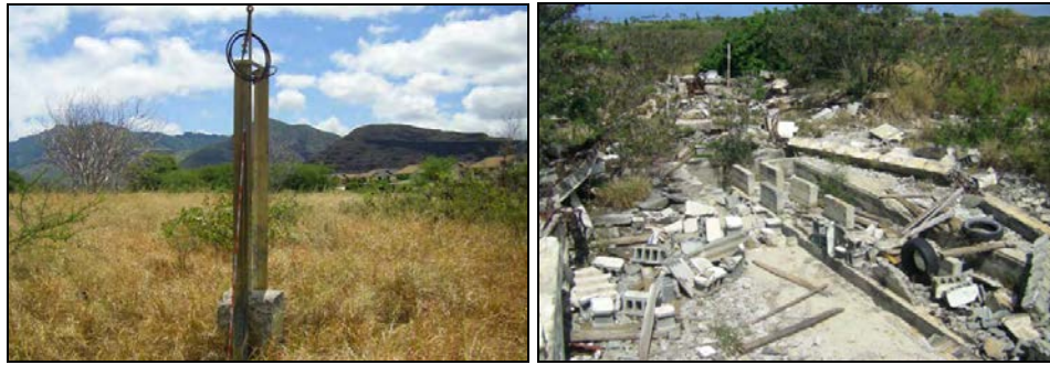
Figure 5. Lualualei antenna foundation system and ruinous station (source: Reith 2009)
