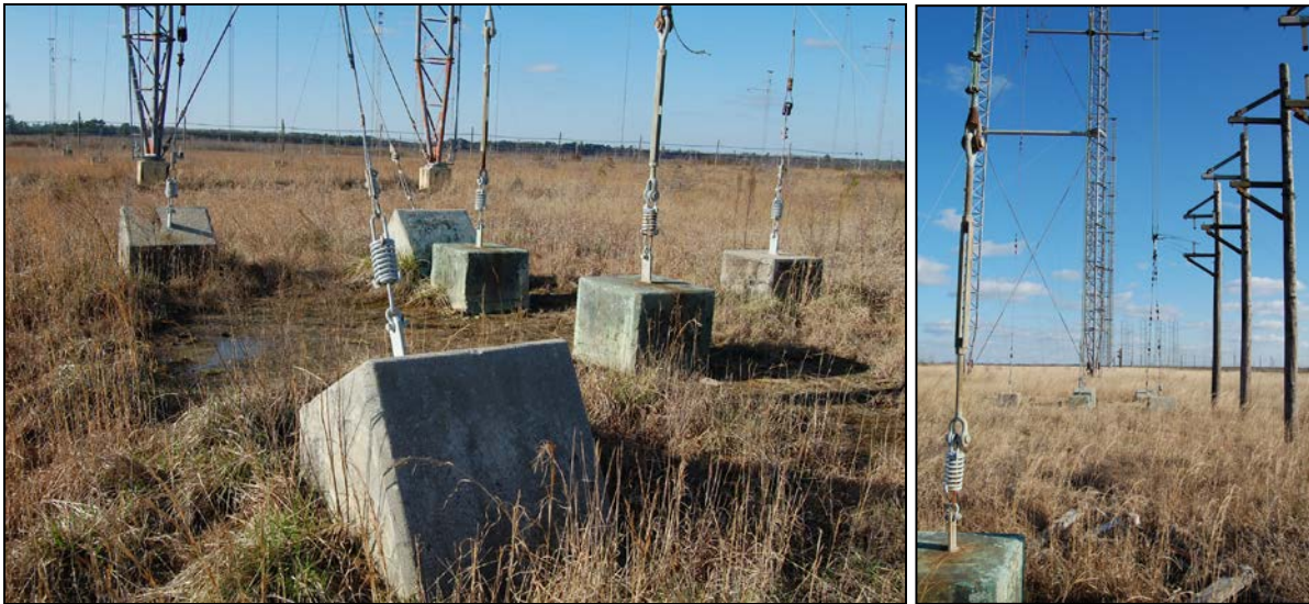
Figure 50. Curtain antenna A-02 anchor piers and guy wires
