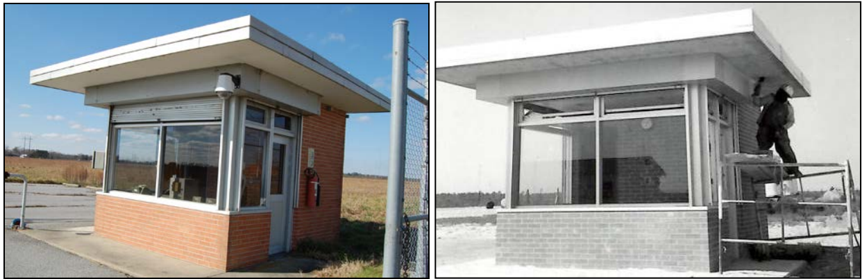
Figure 35. Looking northwest at guardhouse, at left, and building nearing completion, September 12, 1962, at right (both Site A) (source: VOA progress photographs file)
